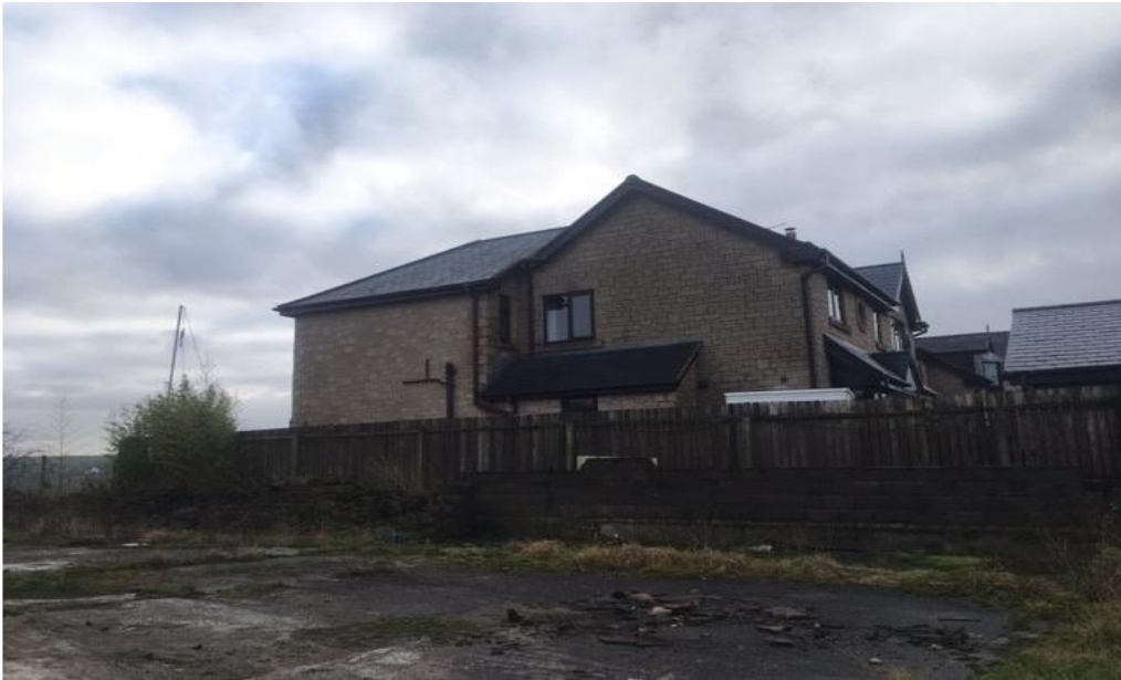
Case officer site photograph, taken 23 rd October 2020 – Gable of No.10 Tower Court, first floor windows on front and gable.
