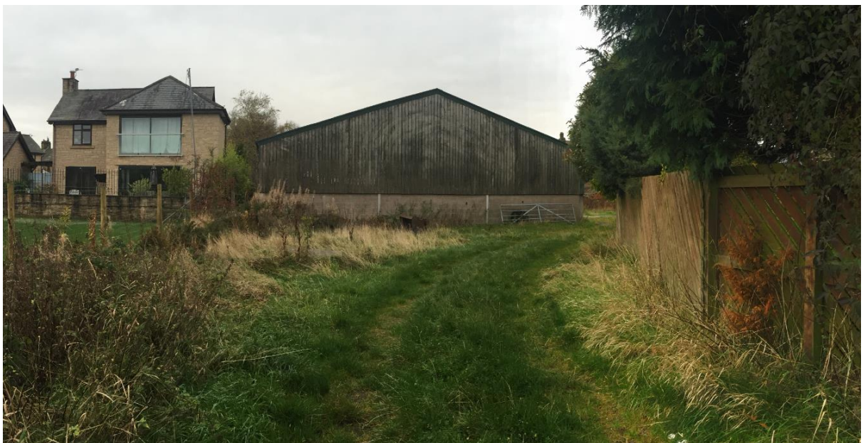
Case officer site photograph taken from the open fields looking towards north-east corner of application site - November 2015
