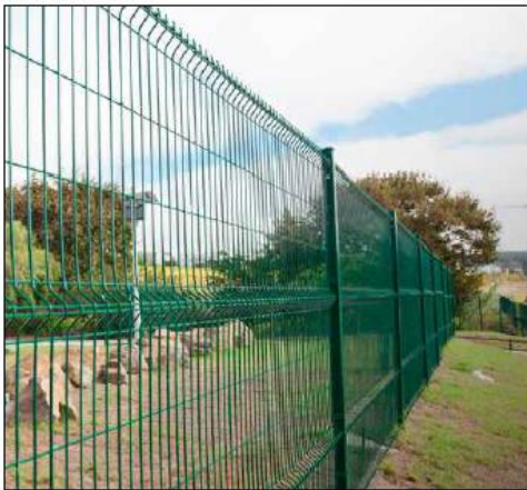
Fig 2: Example of weld mesh fencing
